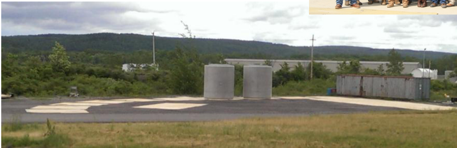
Vertical Storage Casks Placed onto Temporary Storage Pad to Cure
