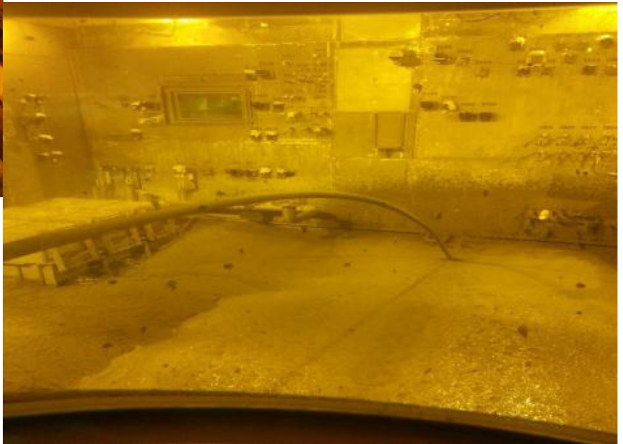
Vitrification Cell Grouting in Progress
