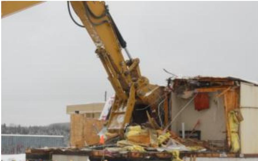
Test and Storage Building Trailer Demolition
